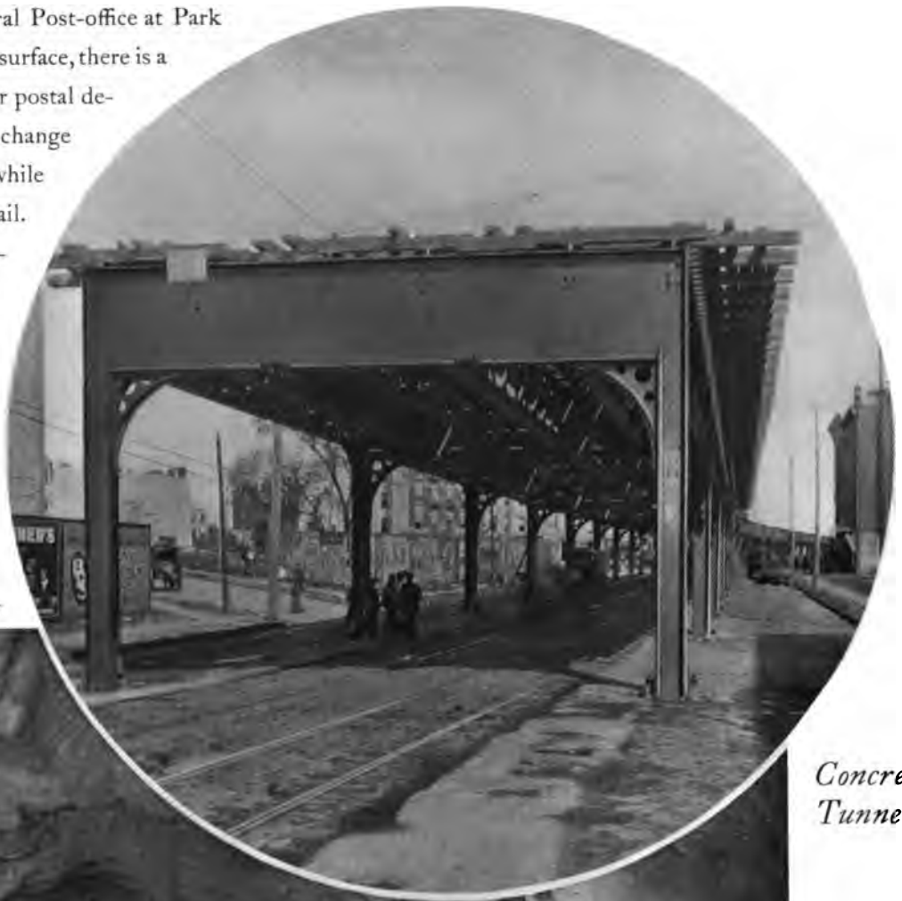
TWO COLUMN BENT VIADUCT
